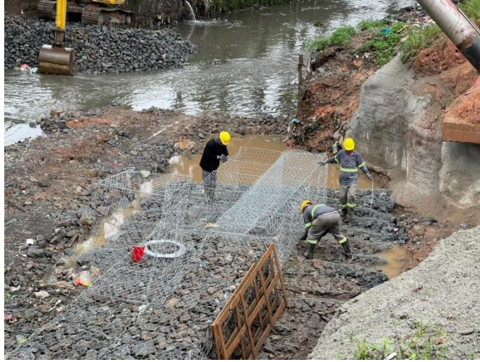
Figure 44. Assembly of gabions.
