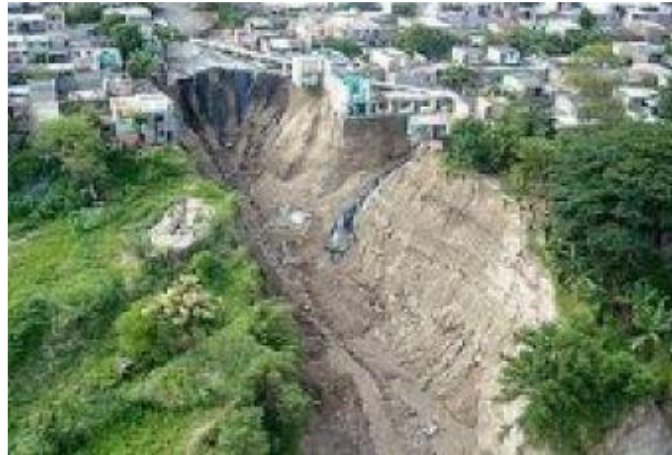
Figure 2. The erosive process caused by tropical storm "Agatha."
