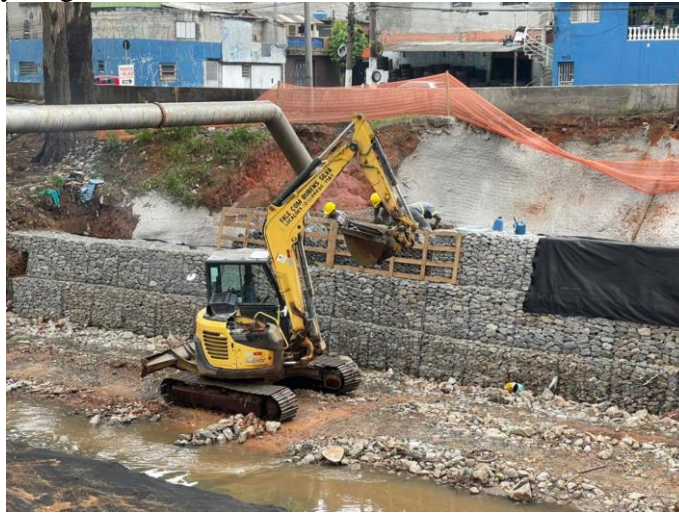
Figure 45. Gabions being filled with rocks
