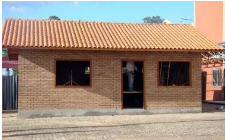
Figure 7. House model using C&DW recycled material.
