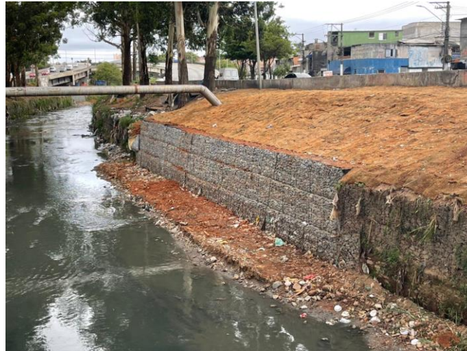
Figure 47. Site #3 after gabions assembling.
