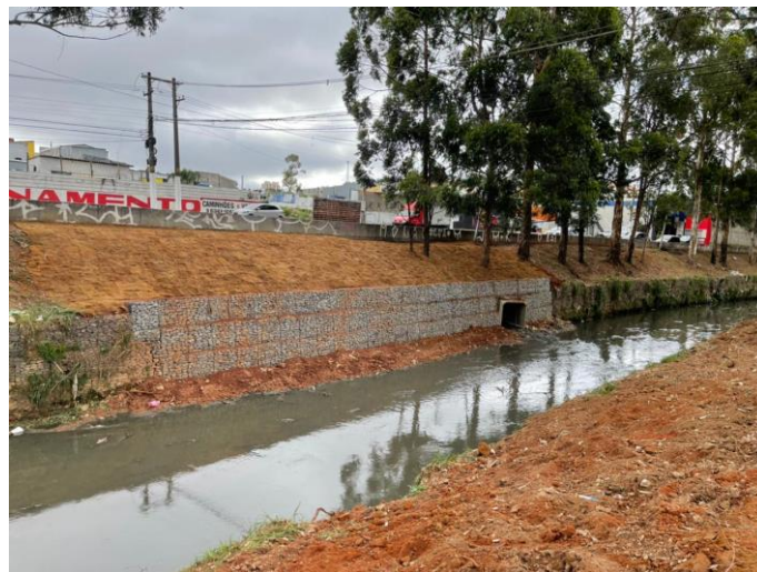
Figure 48. Site #4 after gabions assembling
