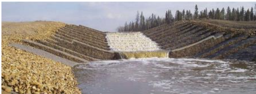
Figure 15. Gabion was used for river cladding. Source: Maccaferri (2020).
