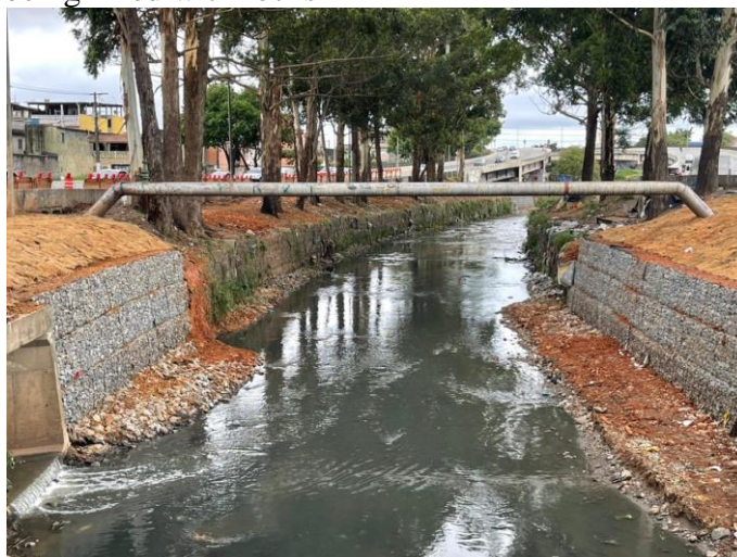
Figure 46. Sites 2 and 3 after gabions assembling.
